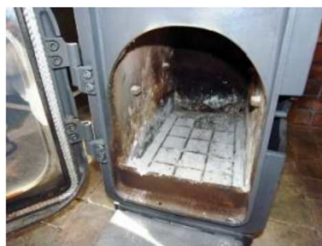
Photo 15: Inside the furnace
