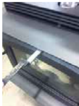
Bypass located above door
